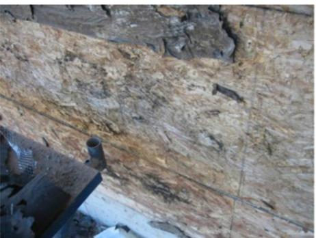
Example: This picture of an out side wooden water soaked wall. Originally it was clad with cultured stone installed incorrectly.
